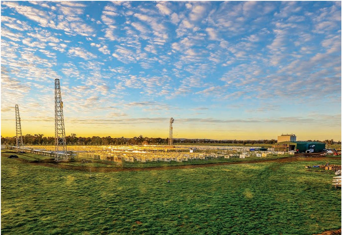
Sunrise during construction of Vast Solar's CSP pilot plant at Jemalong, NSW. The grid-connected plant features thermal storage that enables the delivery of dispatchable electricity, generated with 1.1MW power capacity.
