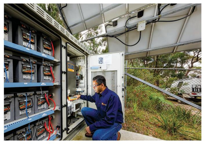
A battery installation at an offgrid telecommunication installation reduced diesel consumption by over 50% reduction through increased generator efficiency.
